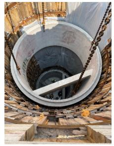
In an effort to expedite construction, Northern Concrete Pipe, (NCP), was contracted to help design and build several 14-foot diameter manholes using 5000 psi
