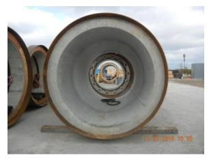
the pipe design to take the project from a two-pass tunnel design, to a one-pass tunnel by installing 60-inch Reinforced Concrete Pipe using a micro tunnel boring machine, (MTBM). This also provided more available water volume that will allow future expansion of their water distribution system.
