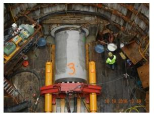
A ¾-inch marine grade plywood joint packer was used as cushion material between the end surfaces of the joints to prevent stress concentrations during the tunneling operation. This joint cushion distributes the axial force preventing point loads on the joint and minimizing potential joint damage.
