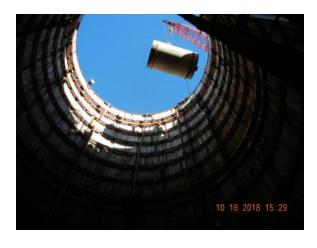
The launching platform shaft, used to push the pipe being installed, is 30-feet in diameter and 67-feet deep. Divers will be utilized to retrieve the equipment once the pipe has been micro tunneled into place.
